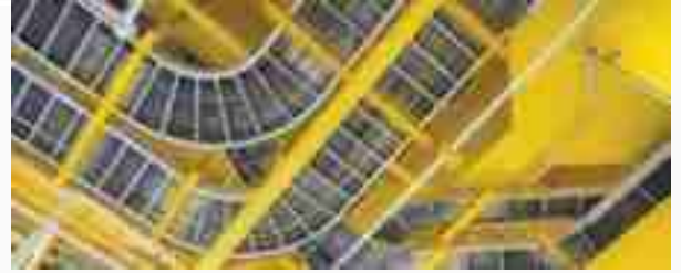
PERMANENT CONSTRUCTION CABLE TRAY
